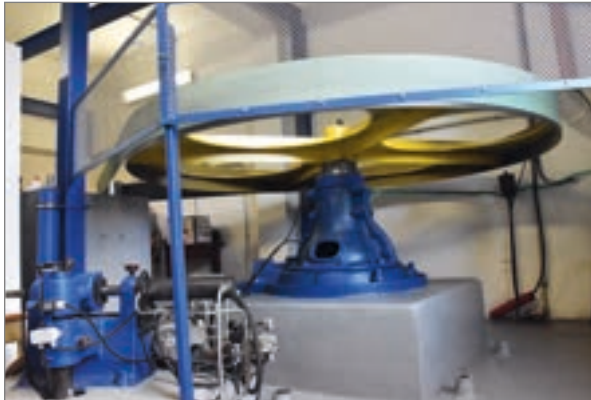
Historically valuable parts are well maintained
