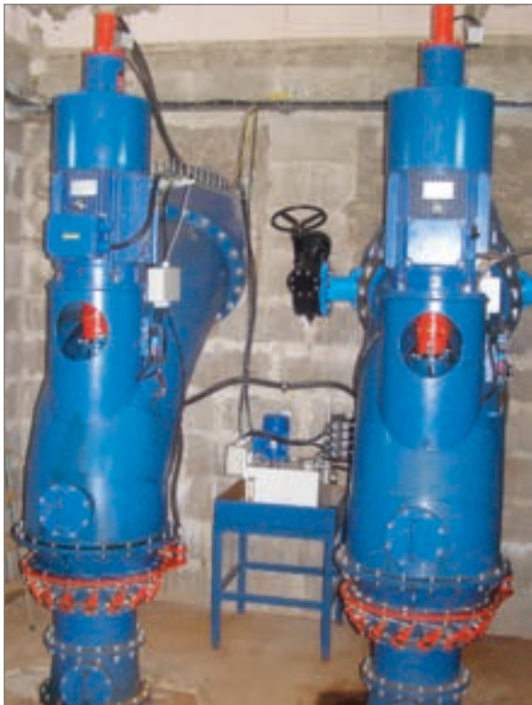
The Kaplan turbine now produces electricity even in the smallest SHPs
