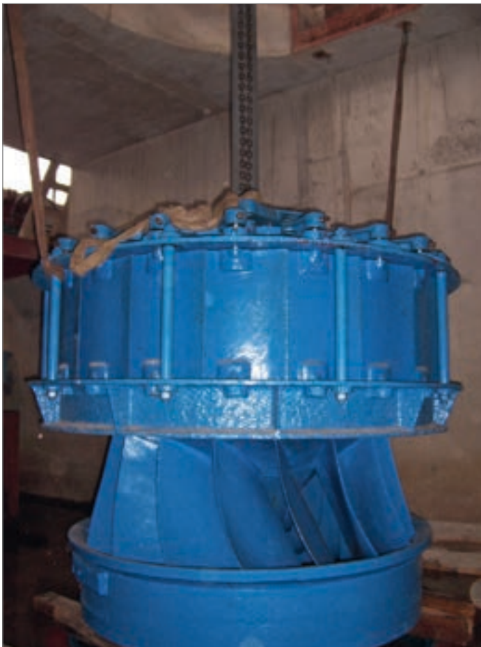
Repairable turbines were being brought back into operation
